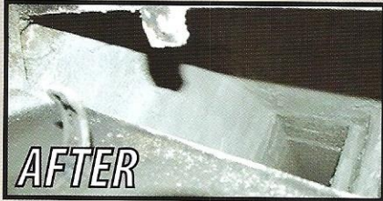
HeatShield Cerfractory Foam Application Seals Gaps, Cracks, Holes, and Streamlines Smoke Chamber Walls
