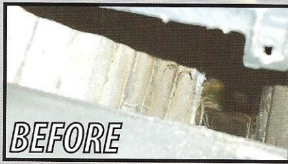
Exposed Brick Corbells Before HeatShield Cerfractory Foam
